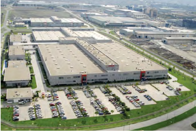
Boshch Diesel Injector Production Facilities - Bursa
