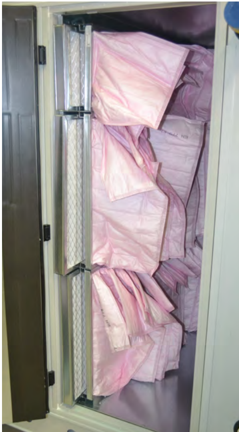
Side withdrawable combined filter (panel + bag)
