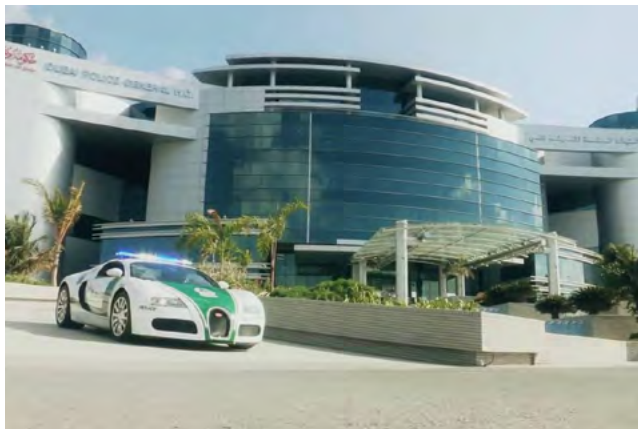
Siemens Headquarters, Dubai - UAE
