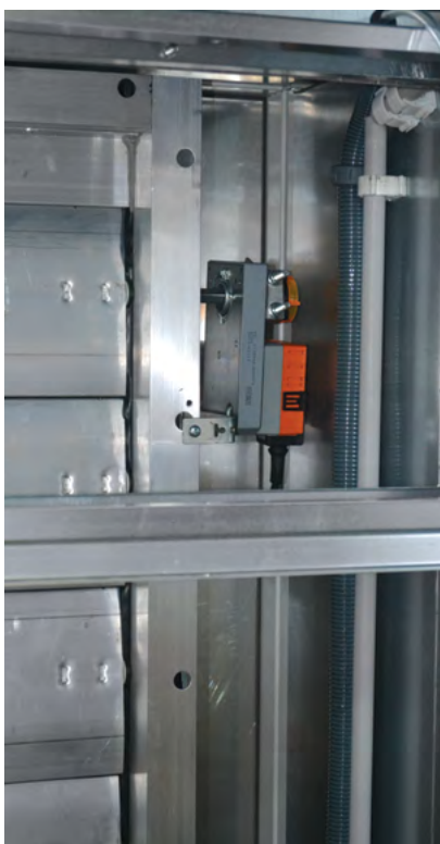
Opposite blade damper with full face opening from front
