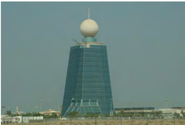
Etisalat Data Center, Fujairah - UAE
