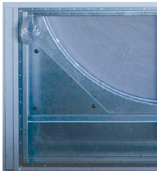
Wheel inspection port
