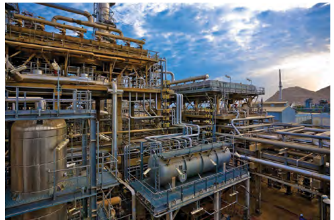
Sohar Refinery - Oman
