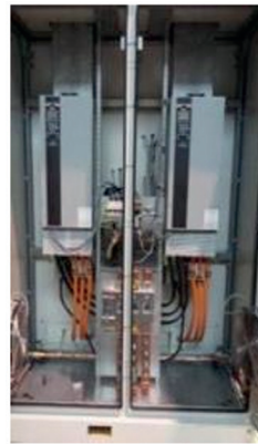
Compressor drives + main power connection
