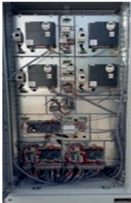
Fan drives + Pump drives + electronic boards
