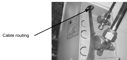
Detail of electrics box supply
