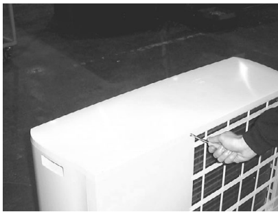
remove the middle screw (rear section)
